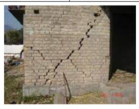
Photo 9: Diagonal cracking of solid wall (Bed joint sliding mode)
