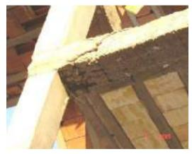
Photo 20: Shear crack in beam near to support
