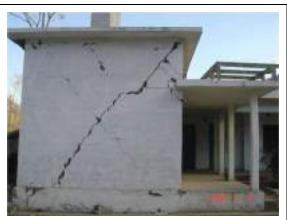
Photo 8: Diagonal cracking of solid wall
