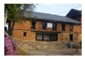
Fig 1.5 (a) Stone in Mud in Ground Floor and Brick in Mud in First Floor
