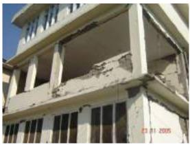
Photo 24: Extreme Damage to Infill wall
