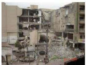
Collapse of ground floor or parts of the building
