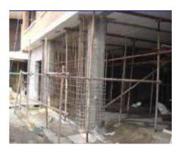
Fig 10. (b) Addition of Shear Wall and Column Jacketing
