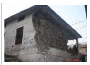
Photo 11: Delamination of outer stone masonry wall
