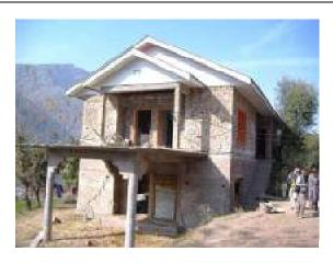
Large and extensive cracks in most walls, roof tiles detach, tilting or falling of chimneys, failure of individual non-structural elements such as partition/ gable walls. Load carrying capacity of structure is partially reduced.
