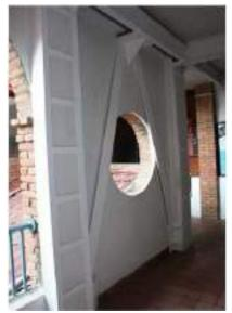
Fig. 11. Retrofitting by Diagonal Steel Bracing
