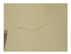
Fig 2.11 Problem due to Crack in Brick Wall
