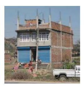
Fig 1.3 Non Engineered Reinforced Concrete Moment Resisting Frame Buildings
