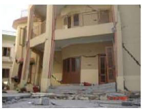
Gaps occur in walls, walls collapse, partial structural failure of floor/ roof, Building takes a dangers state.
