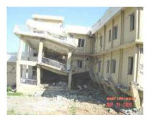
Photo 18: Earthquake damage due to soft story
