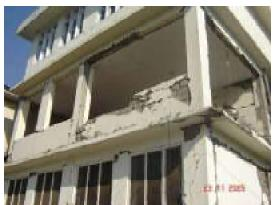
Cracks in column and beam at the base, spalling of concrete covers, buckling of steel bars, Large cracks in partitions and infill walls, failure of individual infill panels Cracks in wall need grouting, architectural repairs required, Seismic strengthening advised
