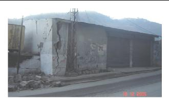
Large and extensive cracks in most walls, roof tiles detach, tilting or falling of chimneys, failure of individual non-structural elements such as partition/ gable walls. Load carrying capacity of structure is partially reduced.
