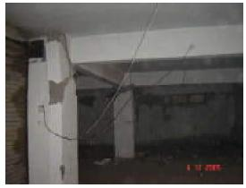
Large cracks in structural elements with compression failure of concrete and fracture of rebars, bond failure of beam bars, tilting of columns, collapse of few columns or single upper floor
