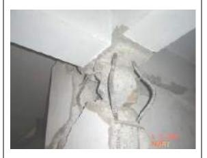
Photo 22: Buckling of column bars
