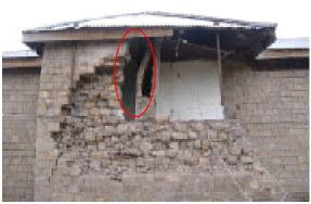
Photo 12: Delamination of outer and inner stone masonry walls
