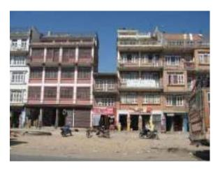
Fig 2.2 (e) Buildings Attached to Each Other Without Seismic Gap (These buildings are liable to suffer in pounding)
