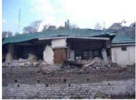
Photo 11: Out of plane failure of block wall
