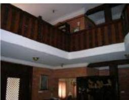
Fig 2.17 (a) Drop in Floor Slab
