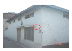
Thin cracks in plaster, falling of plaster bits in limited parts, fall of loose stone from upper part of building in rare cases Building need not be vacated, only architectural repairs needed, Seismic strengthening advised
