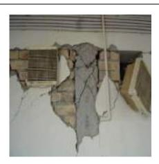
Photo 21: Shear crack in column
