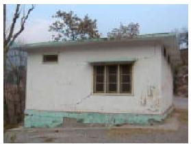
Thin cracks in many walls, falling of plaster in last bits over large area, damage to non-structural parts like chimney, projecting cornices; The load carrying capacity s not reduced appreciably.
