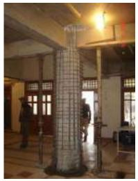
Fig 10. (a) Jacketing of RC Column
